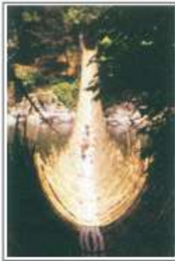
Figure 6.7 : Rope Bridge (Arunachal Pradesh)
